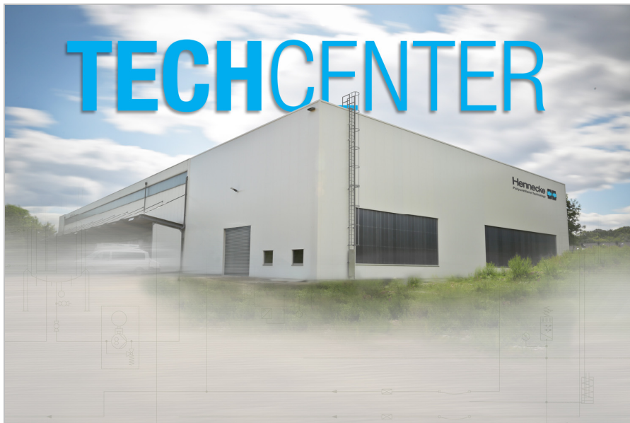
State-of-the-art polyurethane processing technology across a surface of more than 1,000 m 2 : Hennecke's new TECHCENTER
